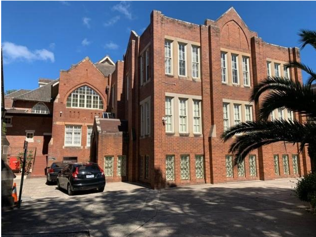
Figure 6: The former St. Paul's rectory extension, viewed from within the site, looking east
