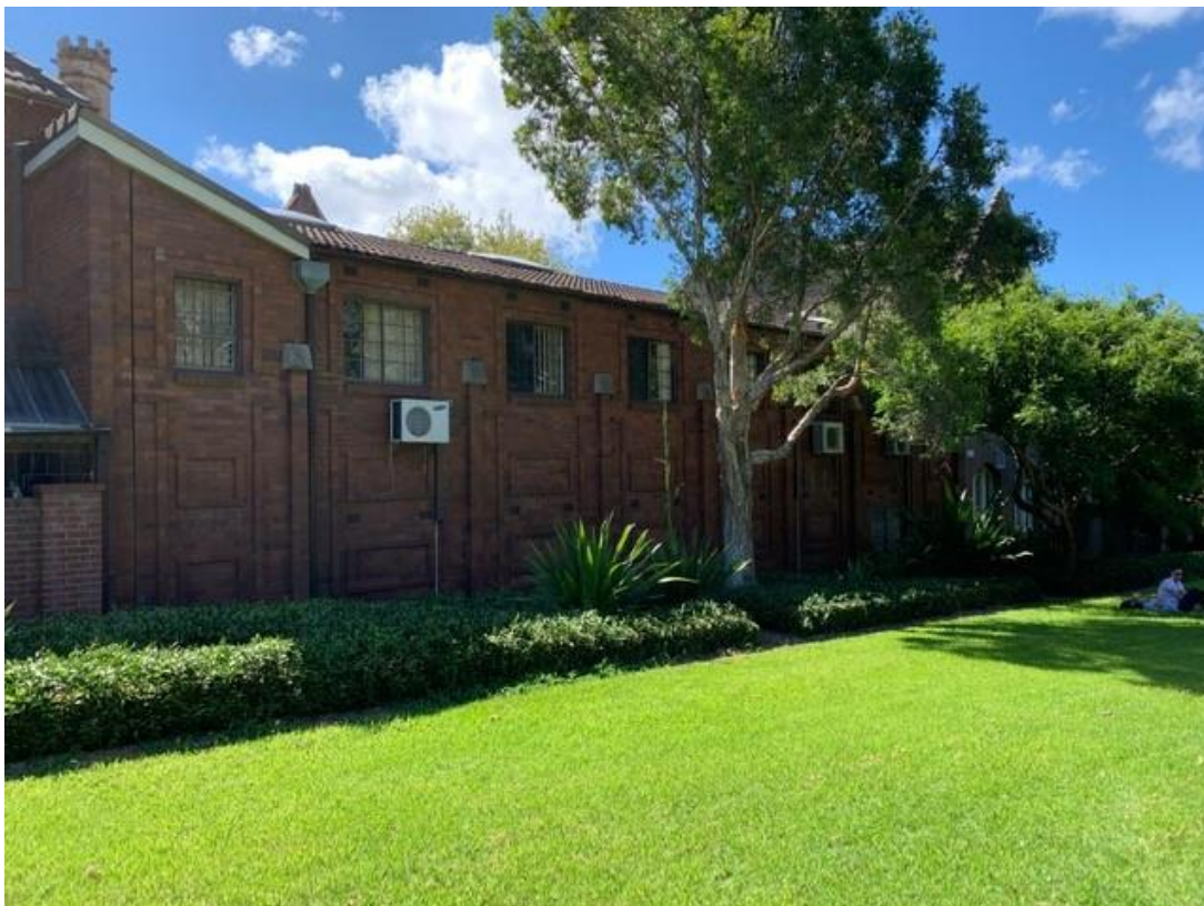
Figure 7: Function Hall, viewed from Prince Alfred Park, looking west
