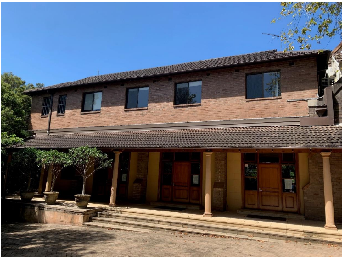
Figure 9: Parish Hall extension, viewed from within the site, looking east
